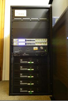
Amplifier and Audio Processing Rack. Via relay control on the Electrovoice DC-One, the Church speakers can be quickly switched from portrait to landscape orientations.
